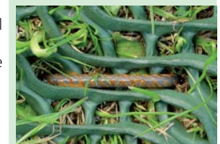
Secured with U-pins
