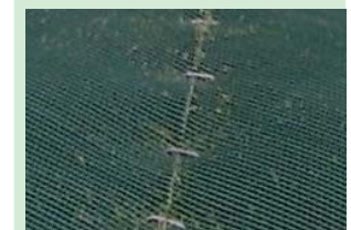
Mesh 'Butt' joined using U-pins
